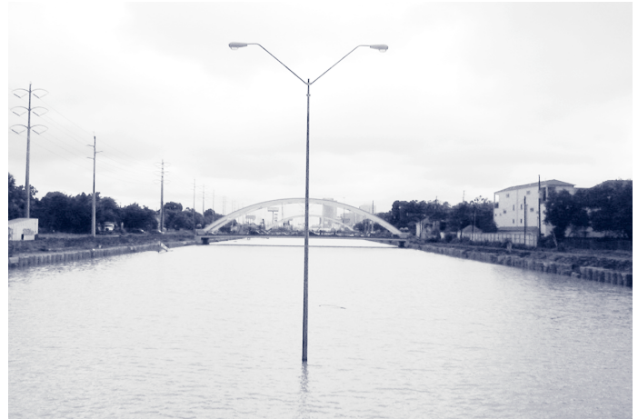
FIGURE 2. U.S. Highway 59 North, heading towards downtown Houston, was covered by flood waters following Tropical Storm Allison
