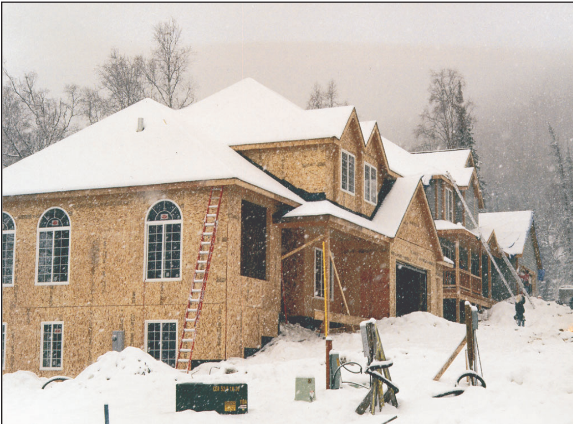
Photo 19: Residential construction site in southcentral Alaska
