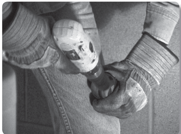
Solution: Using wire brush with power driver
