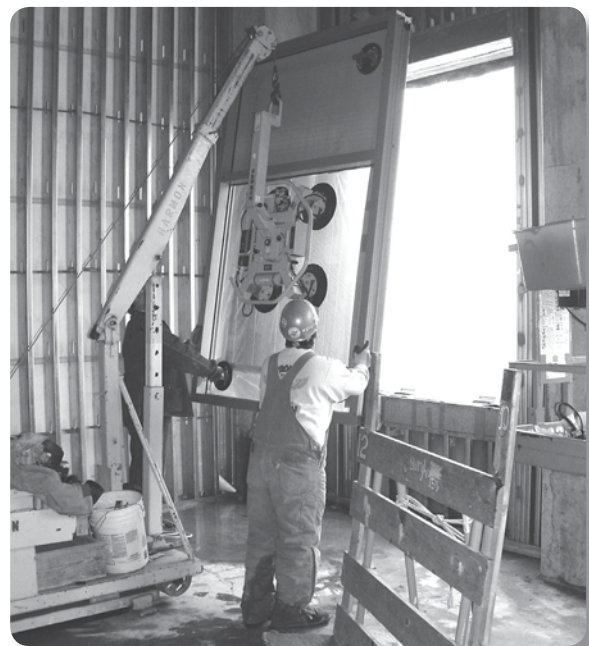
Power vacuum lifter avoids manual lifting
