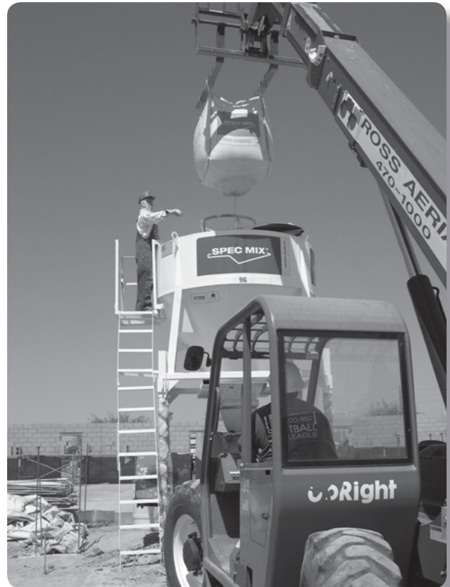
Solution: Loading a silo system
