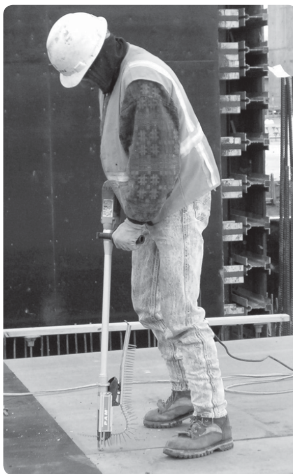
Solution: Autofeed stand-up screw gun
