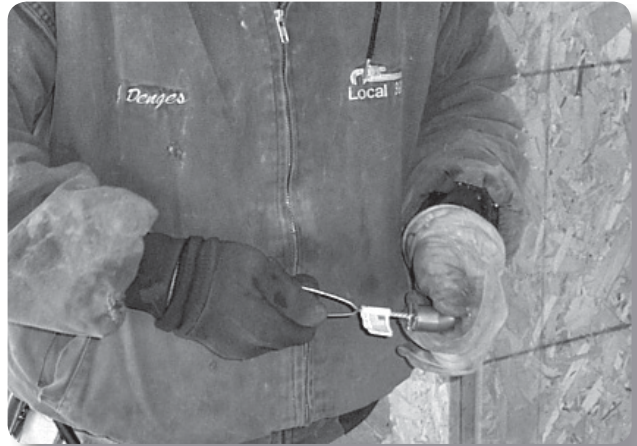
Problem: Brushing copper tube by hand
