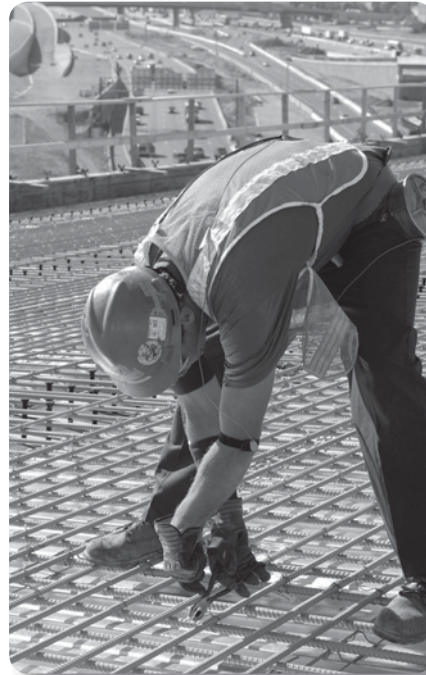
Problem: Tying rebar by hand
