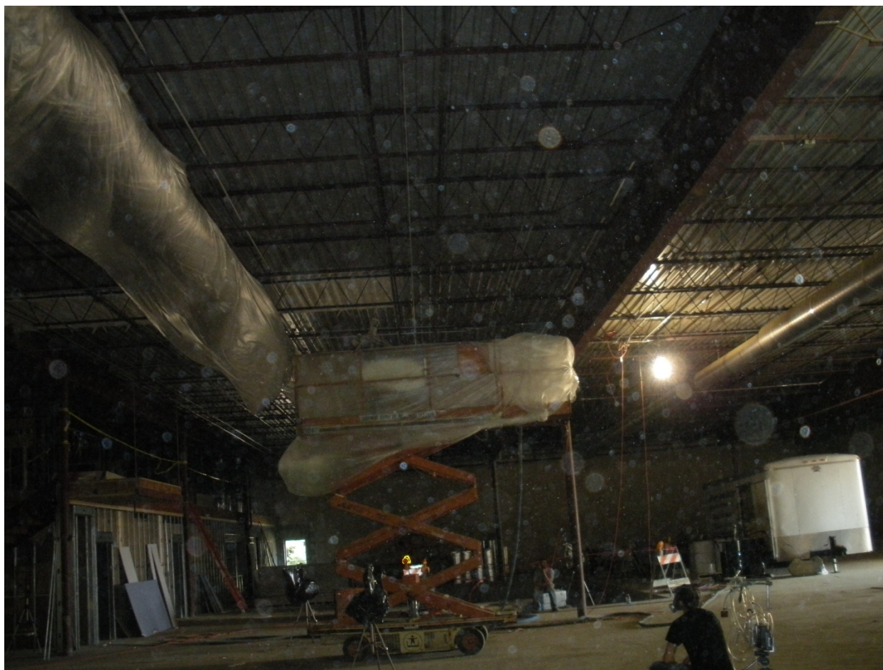
Figure 1: Sprayer applying SPF to the ceiling using a scissors lift
