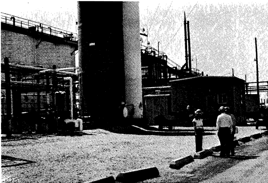
Figure 1. Road separating formaldehyde (on left) and sulfuric acid units. Formaldehyde storage and blending area.
