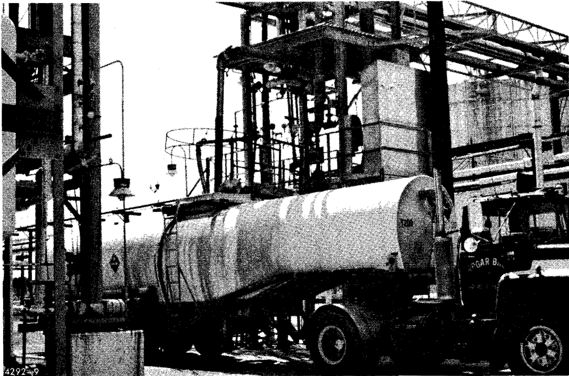
Figure 8. Truck loading area.
