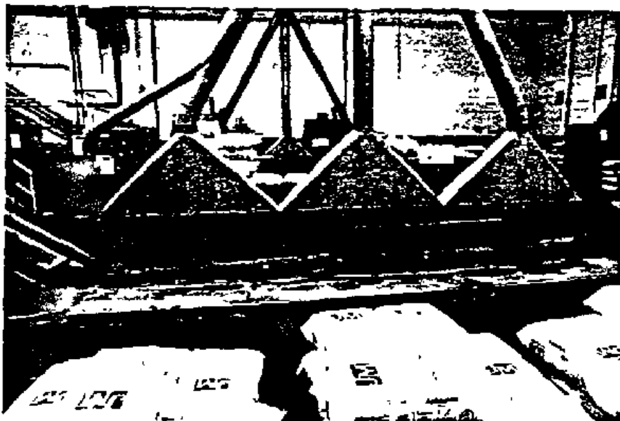
Figure 8. Slot hood next to loading Conveyor. There is a slot hood beneath the transfer point for the loading conveyor and the inclined conveyor which transports the bags to the bag opening machine.
