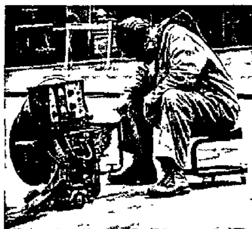
Figure 10 Worker running automatic welder while on stool
