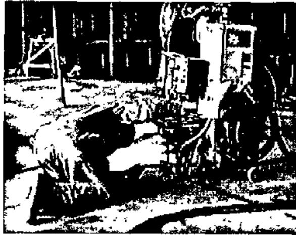
Figure 7 Worker setting up semi-automatic wire-feed welder
