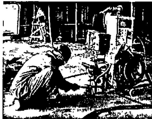
Figure 8 Worker operating semi-automatic wire-feed welder
