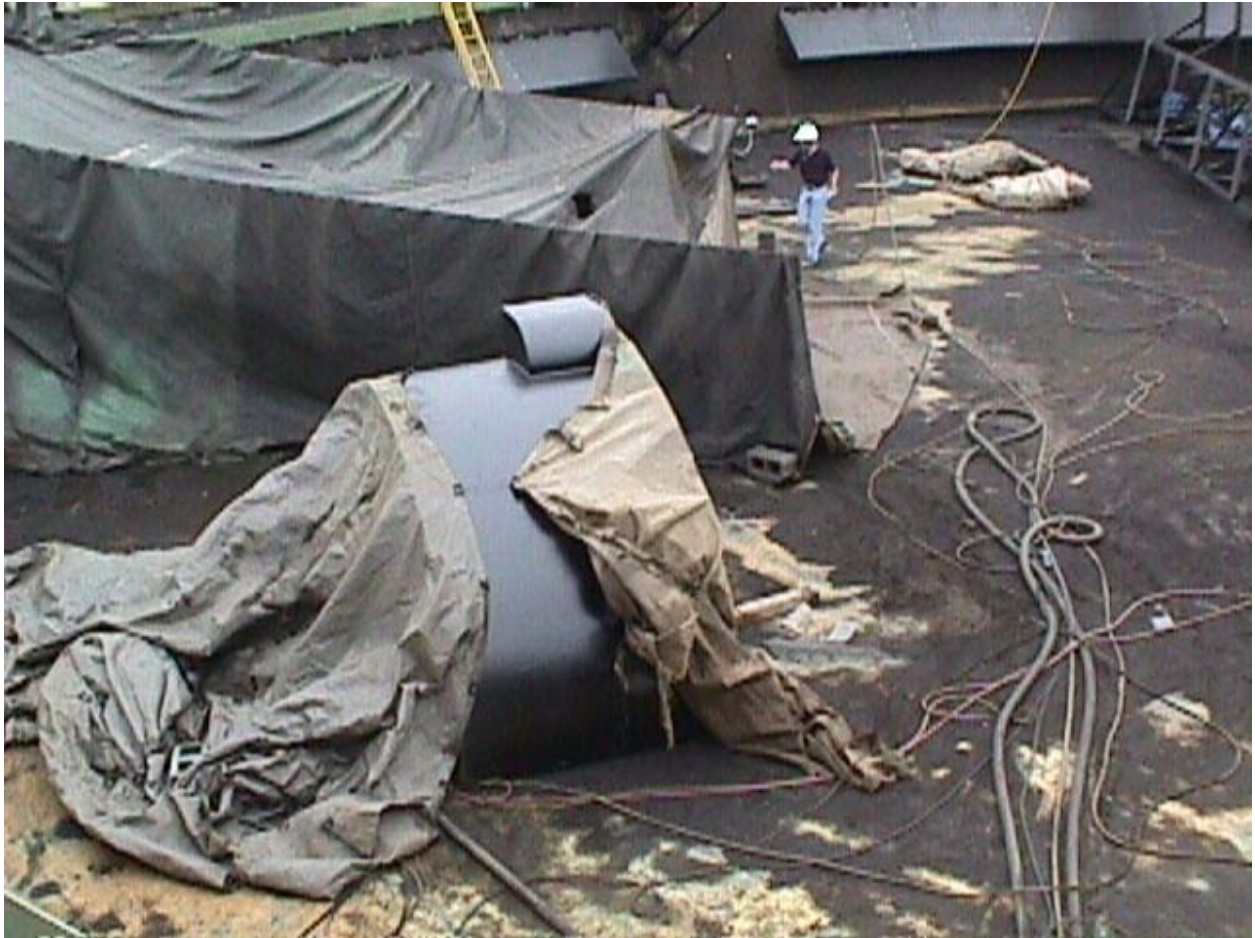
Figure 2. Containment tarps in place for abrasive blasting.
