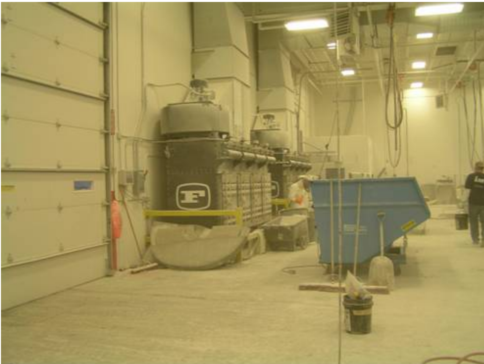
Figure 2: Exhaust ventilation in the web cut and trim area of the M Building
