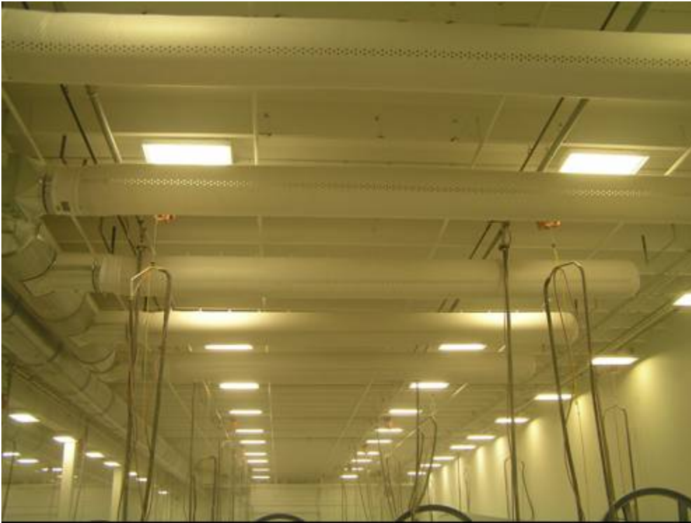
Figure 1: General ventilation supply in the M Building web cut and trim area
