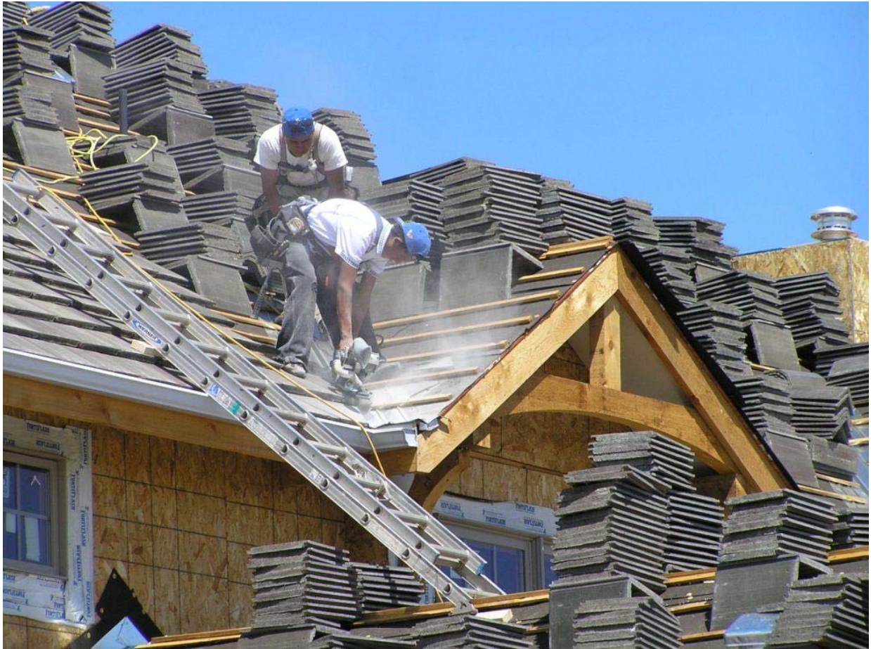
Figure 3. Roof arrangement while installing tiles.
