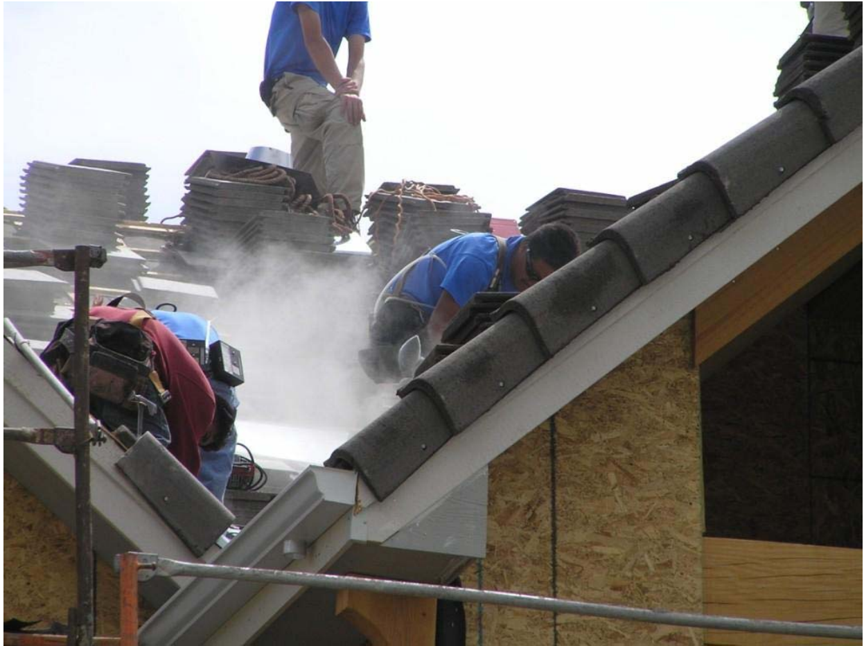
Figure 5. Workers cutting concrete roofing tiles.
