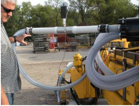
Figure 7 - Exhaust ventilation measured with meter in line
