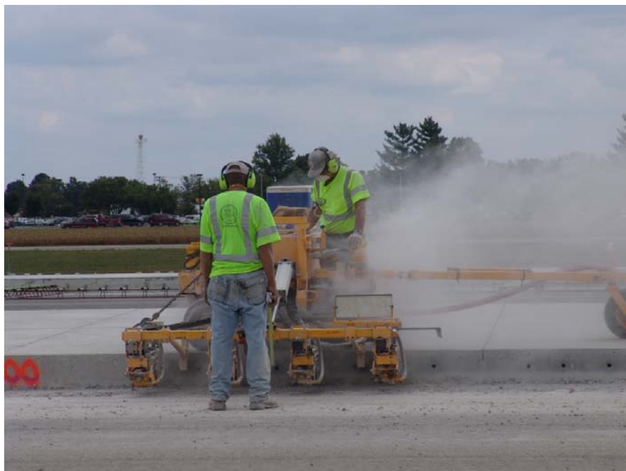
Figure 2 - Laborer Operating an E-Z Drill Dowel Drill
