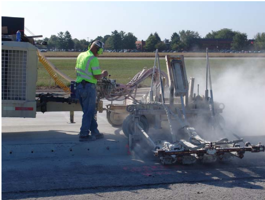
Figure 1 - Laborer Operating a Minnich Dowel Drill
