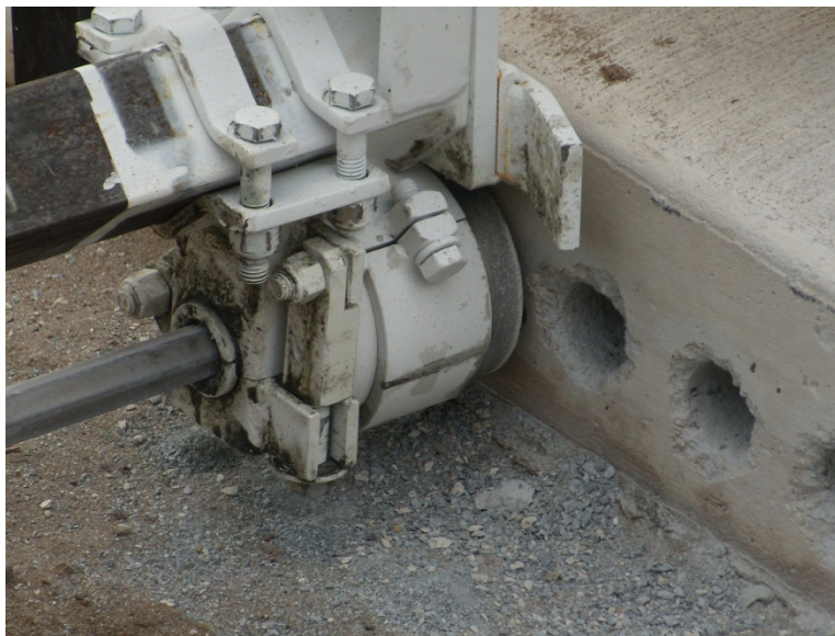
Figure 3 – Hood Surrounding Drill Steel at Concrete Surface
