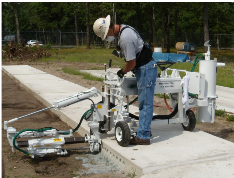
Figure 1 – Laborer Operating Dowel Drill
